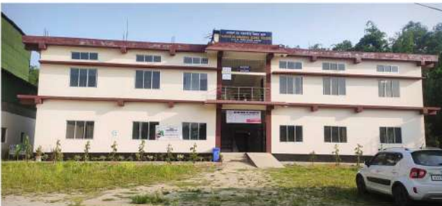
Narayan Chandra Borgohain Science Building
